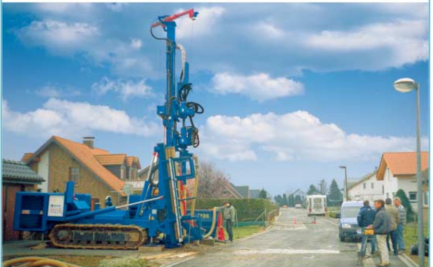
Drill rig type HBR 205 GT
