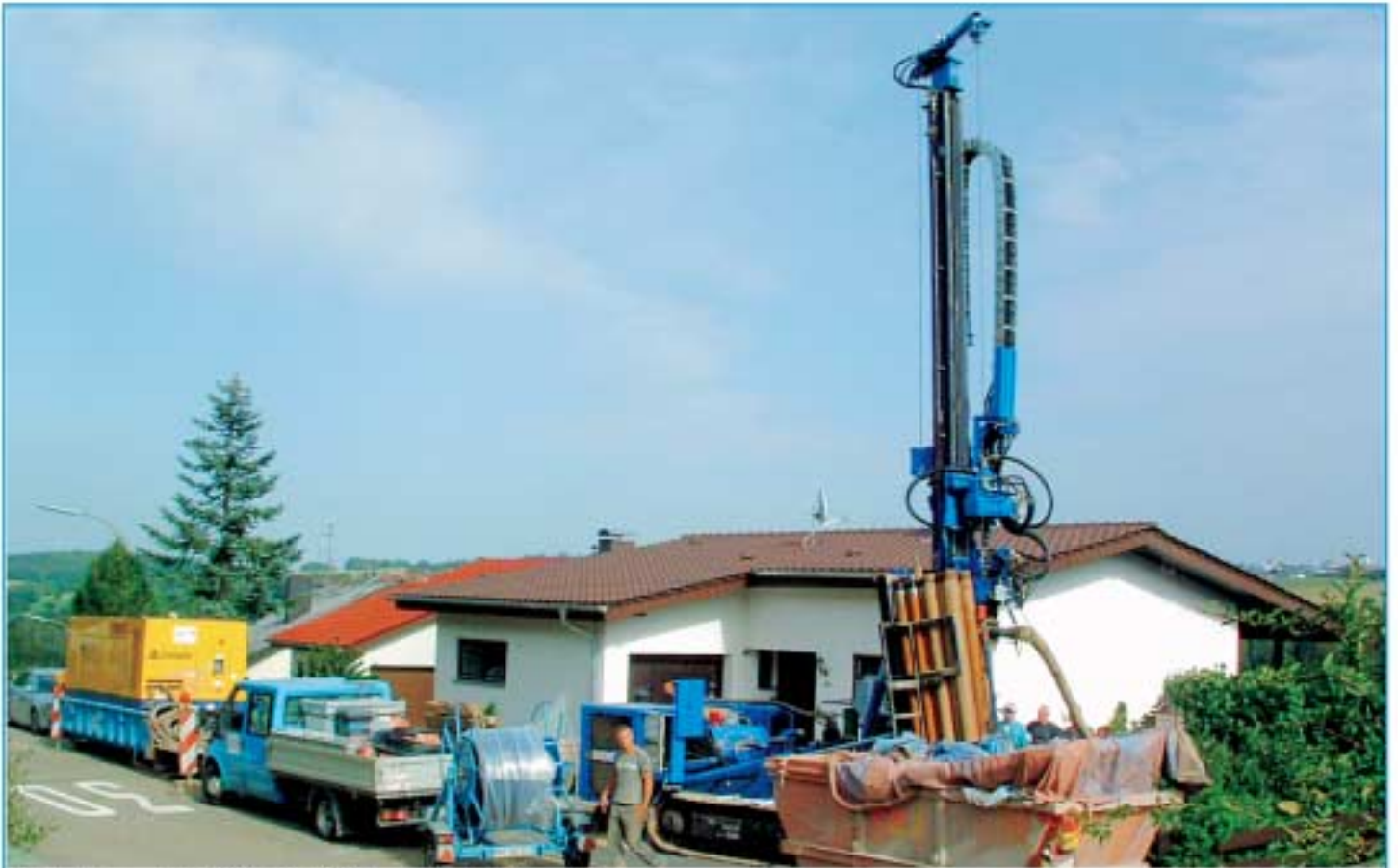
Drill rig type HBR 205 GT, 20 t pull back drill mast.
